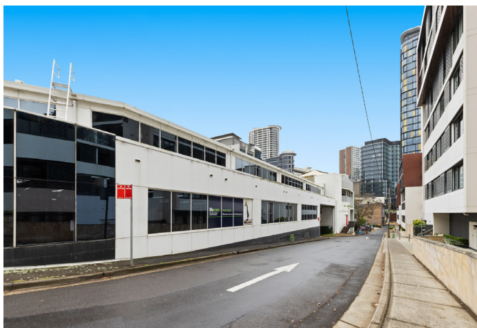
Figure 29: View from Marshall Lane facing east. Source: TZG Heritage, 2025.
