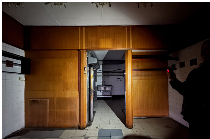
Figure 36: Bakery fitout. Source: TZG Heritage, 2025.
