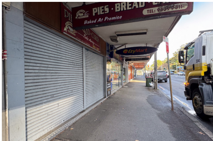
Figure 35: Shopfront - this tenancy is currently vacant. Source: TZG Heritage, 2025.
