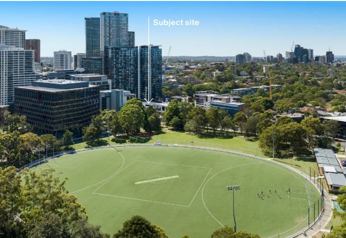
Figure 19: View of Gore Hill Park located northwest of the subject site. Source: Client supplied.
